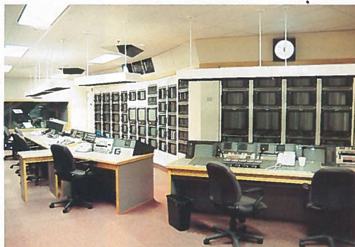
The main studio control centre.
